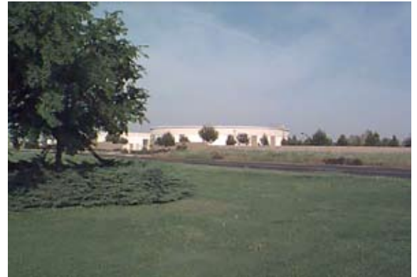
Aesthetic concerns were key in designing this 2-million-gallon ground-level tank, which is close to mixed-use development.
