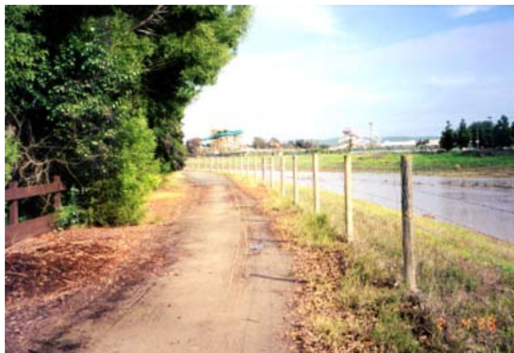
The alignment of Central Contra Costa Sanitary District’s A-Line Interceptor will transverse several sensitive areas, including this trail along the Contra Costa Canal.
