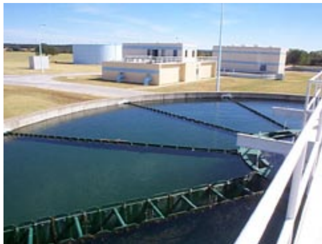
The existing plant will be upgraded with new low-pressure membranes and reverse osmosis.
