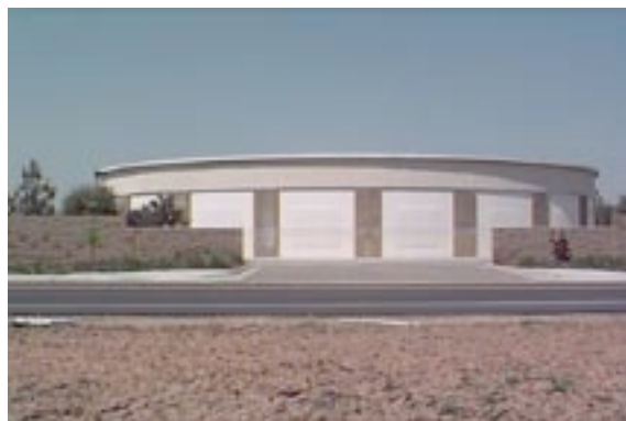
Carollo provided design and construction services for the City of Clovis' largest water storage reservoir.
