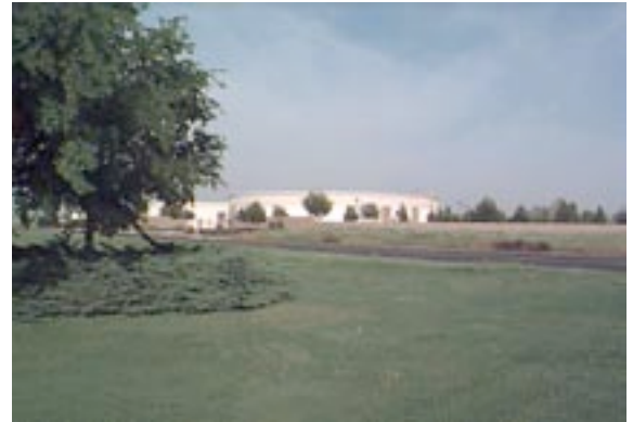
Aesthetic concerns were key in designing this 2-million-gallon ground-level tank, which is close to mixed-use development.
