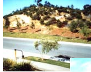
Site after construction. Work involved completely removing the knoll and rebuilding it after reservoir construction.
