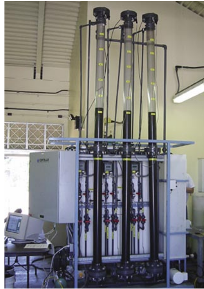
Fixed-bed bioreactors were pilot tested at the Castaic Lake Water Agency.
