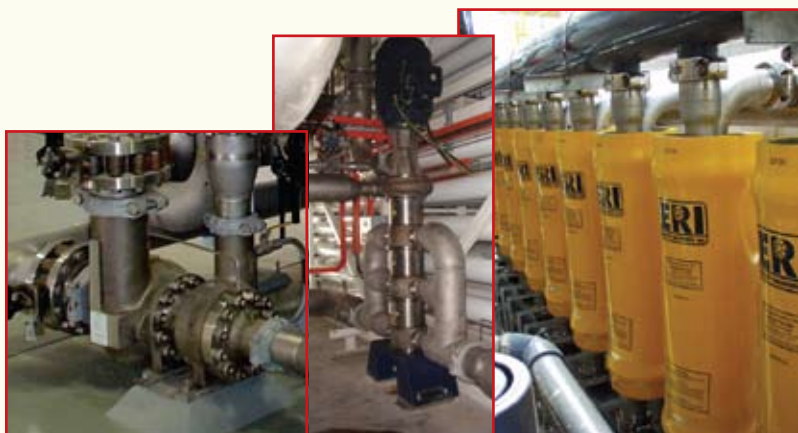
There are two primary types of ERDs used in brackish groundwater RO applications: turbine driven pumps (left and middle) and isobaric devices (right).
