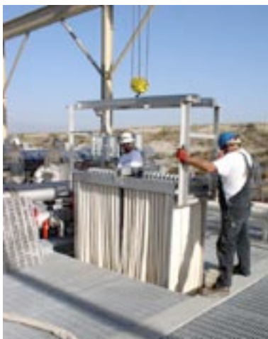
The Redlands Recycled Water Facility employs new technology using immersed MF membranes in a MBR followed by disinfection with sodium hypochlorite.
