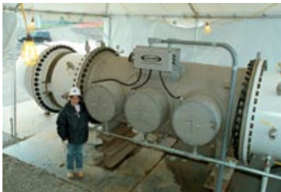
Validation of a 40-mgd UV reactor moves large-scale UV from research to practice.
