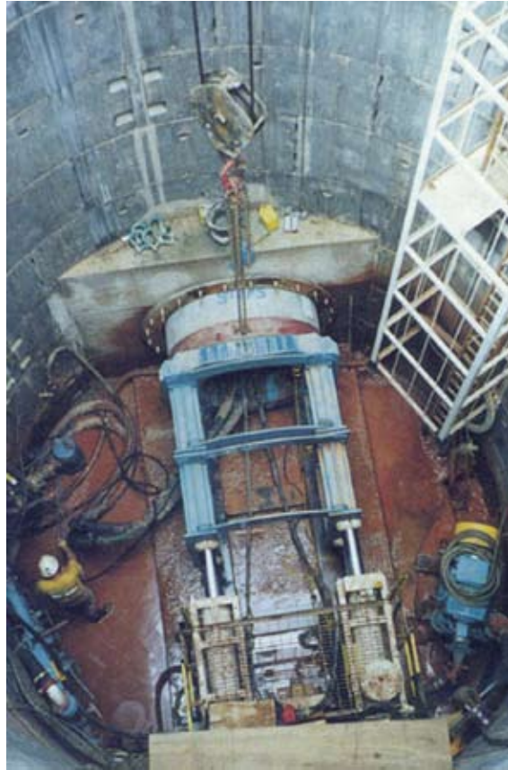
The MTBM used for San Jose's Monterey-Riverside Sanitary Sewer Improvements project featured a pressure-balanced cutting chamber and slurry spoil removal.
