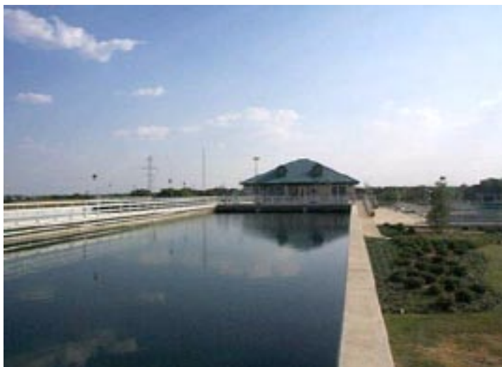
Carollo is designing a second water treatment plant for the Upper Trinity Regional Water District. The new facility will provide additional treatment capacity to UTRWD's service area, which is currently served by the existing regional treatment facility, shown here.
