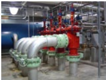
Eight skids equipped with 24 18-inch Aquasource membrane modules help to meet plant production and redundancy requirements at the Lake Forest Water Treatment Plant.
