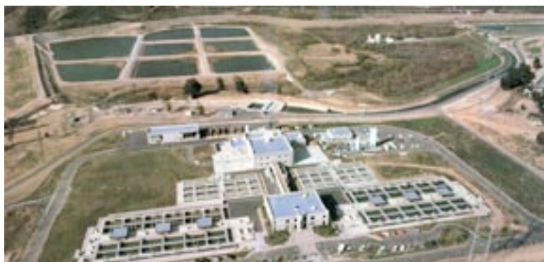
Carollo developed detailed design criteria from bench- and pilot-scale studies that will help the 600-mgd LAAFP address arsenic removal.
