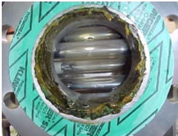
Algae growth upstream and downstream of the medium-pressure UV pilot reactor was an operational issue for the Everglades pilot study. Algae growth is caused by visible light emitted from the medium-pressure UV lamps.
