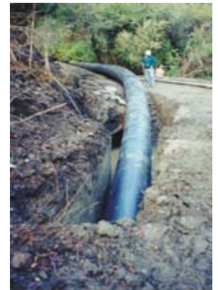
Multiple Diameter Pipe Bursting Project, Hillsborough, California.
