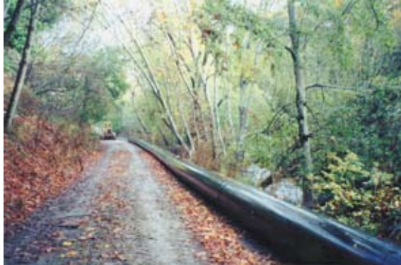
Multiple Diameter Pipe Bursting Project, Hillsborough, California.
