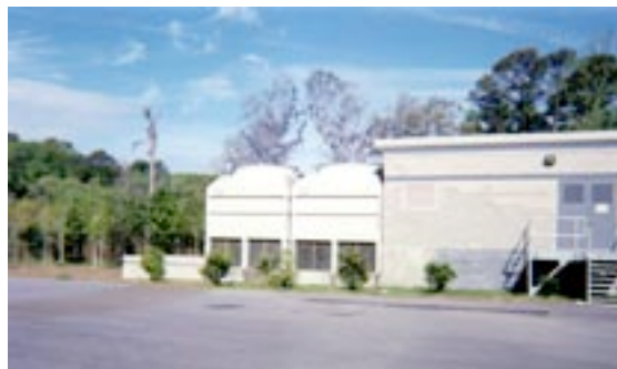
Brackish, geothermal well water is cooled from 122°F to 104°F by a heat exchanger/cooling tower process.
