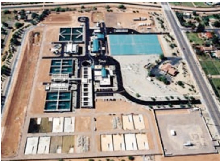
Ozonation and biological filtration will improve aesthetic and health-related water quality for the Town of Gilbert, AZ.
