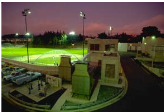
Daly City's underground storage facility below the baseball diamond is one example of the integration of public amenities and a public works project.
