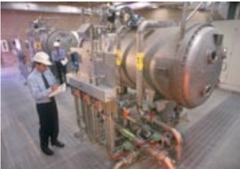
Carollo evaluated ozone and nanofiltration for removing color from the Mesa Consolidated Water District's groundwater supply.
