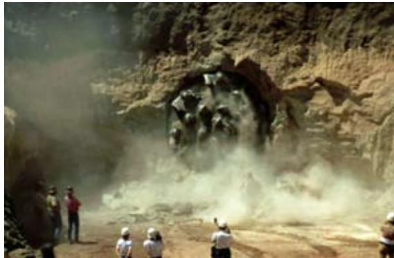
The team managed 20 individual construction contracts including four miles of 12-foot-diameter tunnel bored through the River Mountains.
