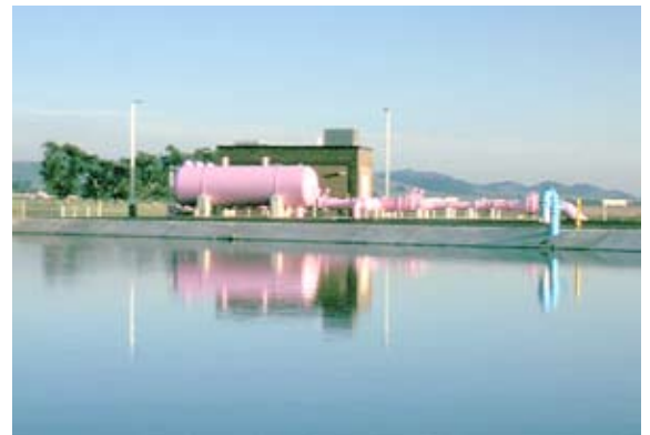
Carollo's design of water recycling facilities for the Napa Sanitation District features cost-efficient distribution pumping and a 20-acre-foot recycled water reservoir.
