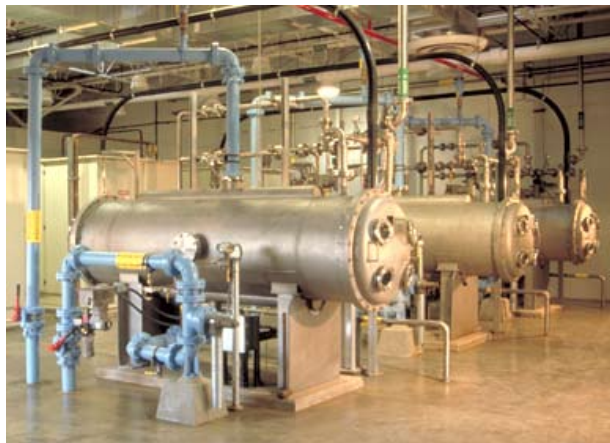
Carollo used computational fluid dynamic modeling at two Arlington water treatment facilities to increase ozone reactor efficiency by 20 percent and significantly reduce construction costs.
