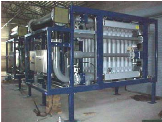
Carollo provided pilot testing, planning design, and construction services to the City of South Bend for the first low-pressure membrane water treatment plant in the State of Washington.
