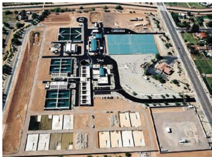
Carollo's design of Gilbert's water treatment facility includes the addition of ozonation to provide primary disinfection and meet future regulatory requirements.
