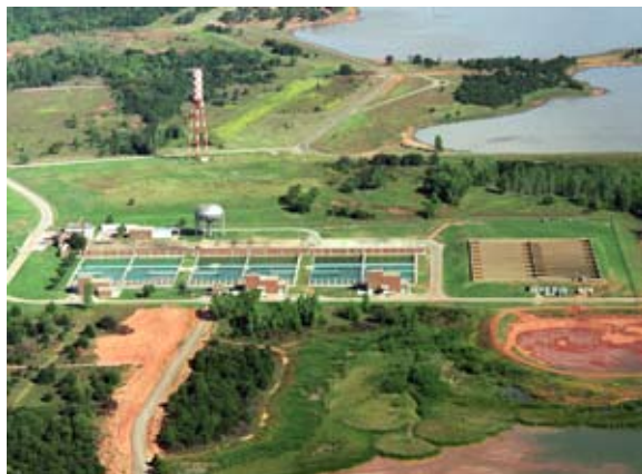
The expansion of Oklahoma City's Draper Water Treatment Plant will result in a savings of $7.1 million through hydraulic improvements and reduced use of existing facilities.
