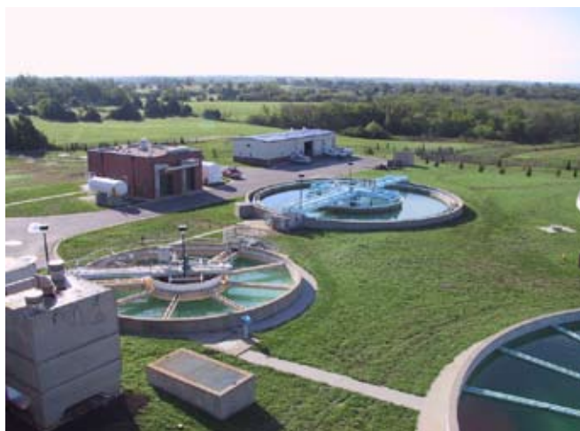
Utilizing existing plant infrastructure at Olathe's Water Treatment Plant No. 2, Carollo developed an innovative plan to meet peak demand without bringing membrane facilities online until months later. This eased a tight schedule and reduced construction costs.
