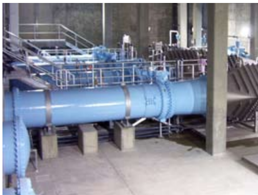
Carollo provided construction services for the installation of large-scale WEDECO K143 reactors validated to flows of 40 mgd.
