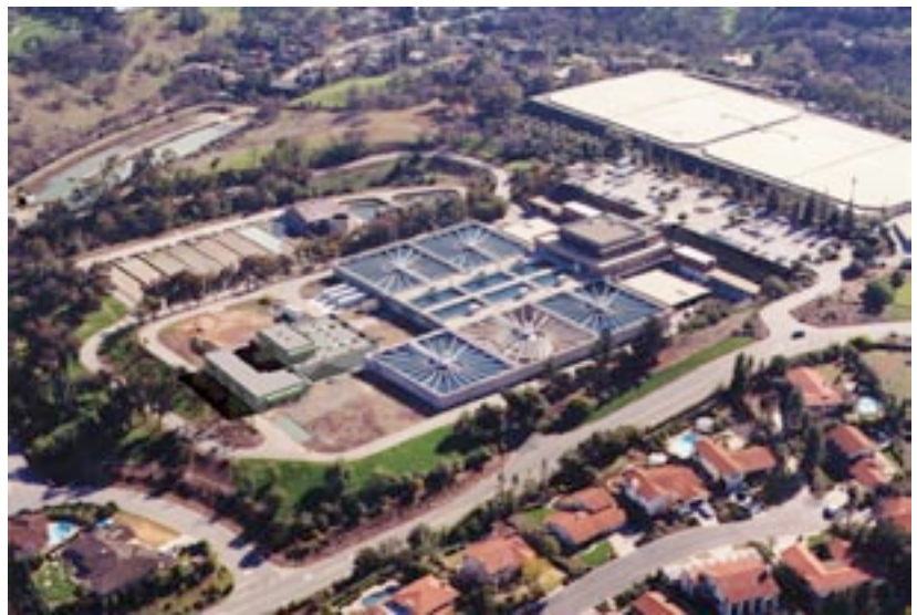
Carollo provided pre-design for 242 mgd of UV disinfection facilities for the Santa Clara Valley Water District's three water treatment plants.
