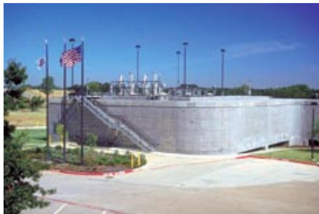
Through the use of computational fluid dynamic modeling, Carollo was able to increase ozone reactor efficiency 20 percent, significantly reducing construction costs.
